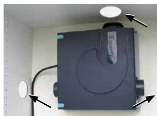
17. Carry out the holes for the passage of the ducts in front of the inlet and outlet sleeves.
