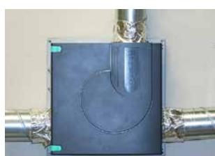
20. Connect the 2 extract units and the extract grille: the fan is ready to operate !
