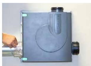
19. Encase the duct then make it integral by using a special AV adhesive.
