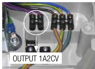
11. Output 12 VAC : Connect if necessary 1 or 2 extract units with peak airflow supply.
